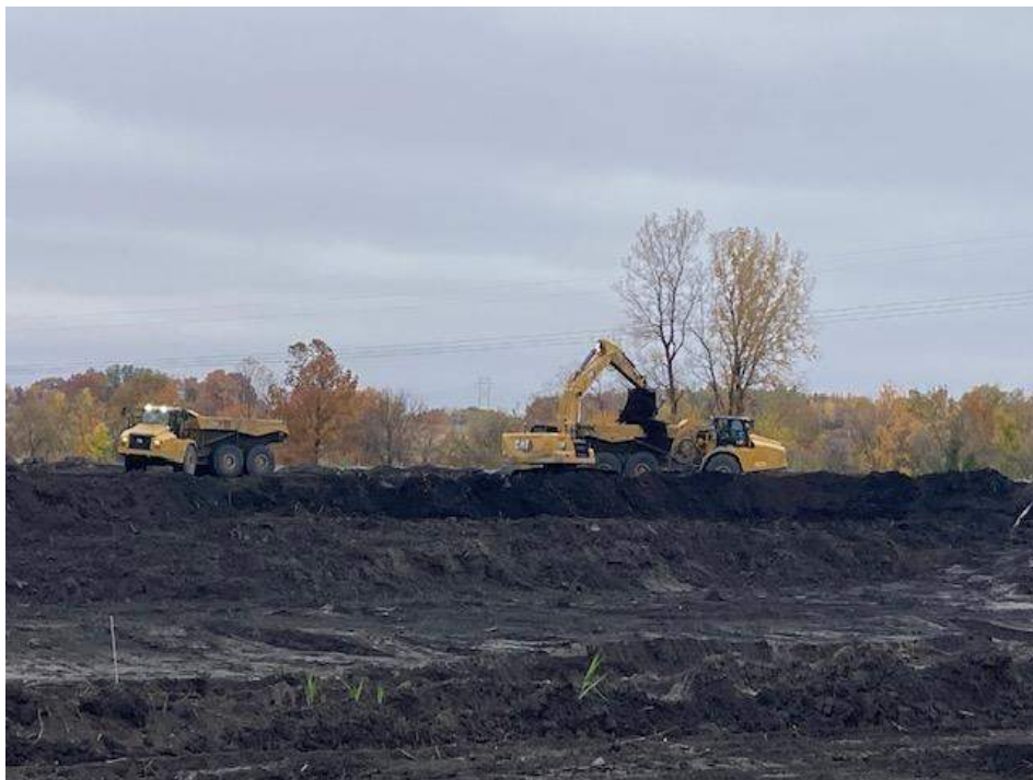
Photograph 8. Loading ash into haul trucks for transportation to landfill.
