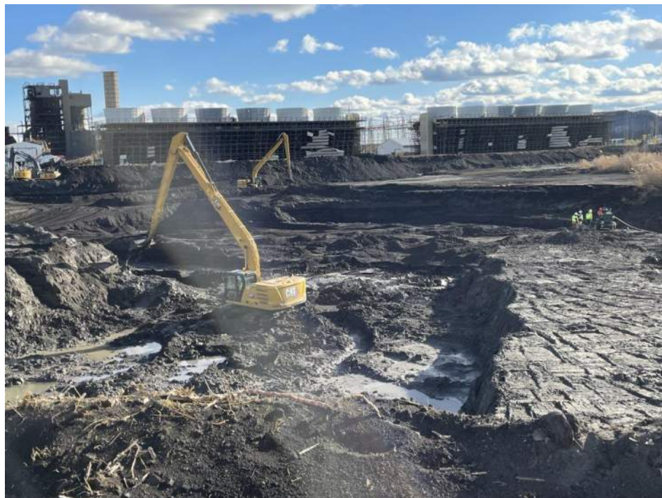
Photograph 14. Lowering rim ditches to continue dewatering ash. (Photograph taken by Charah Solutions, LLC, December 2023)
