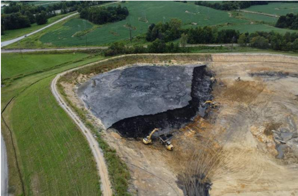
Photograph 39. Excavating and loading ash material from west corner of impoundment.
