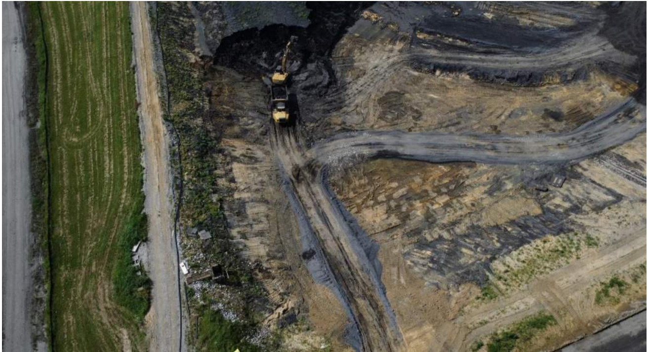
Photograph 31. Loading ash into haul truck for transportation to landfill.
