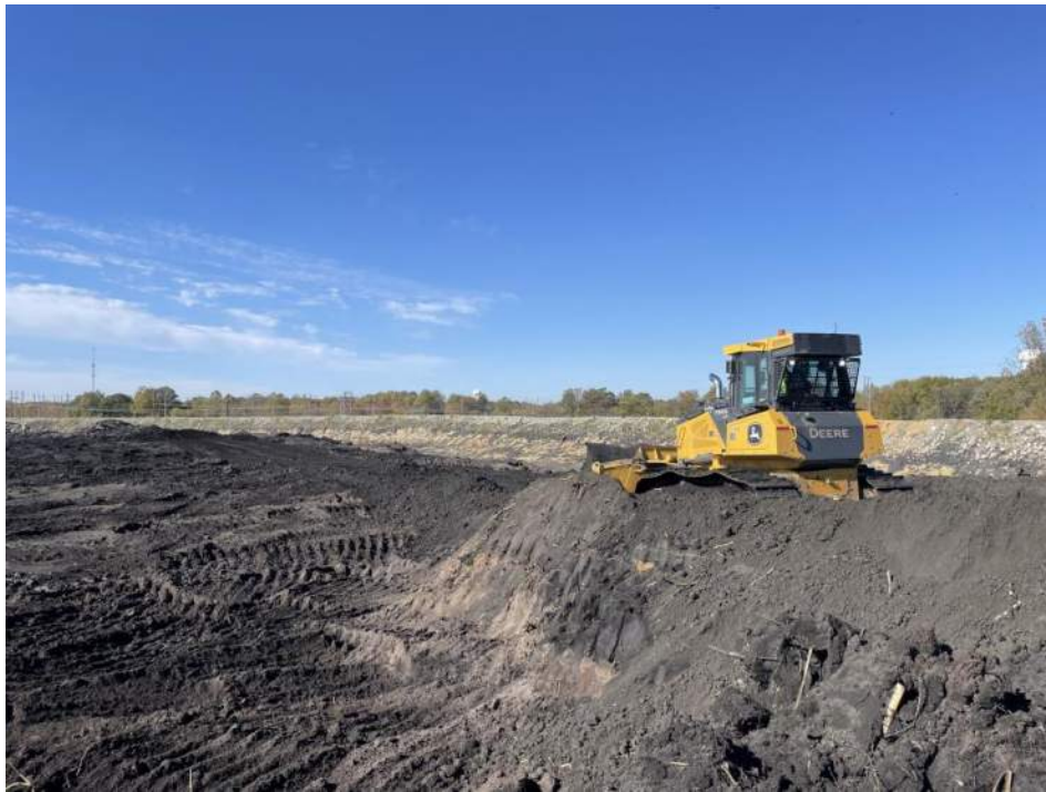
Photograph 7. Bridging over impoundment area to provide work platform for equipment.
