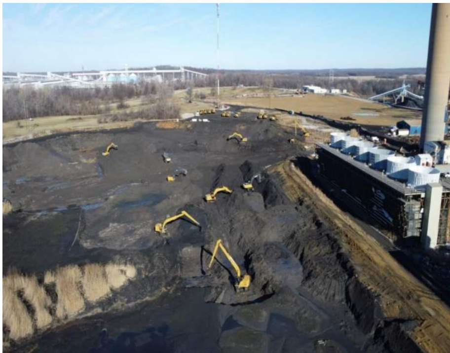
Photograph 18. Material excavation and stockpiling within decant area for dewatering.
