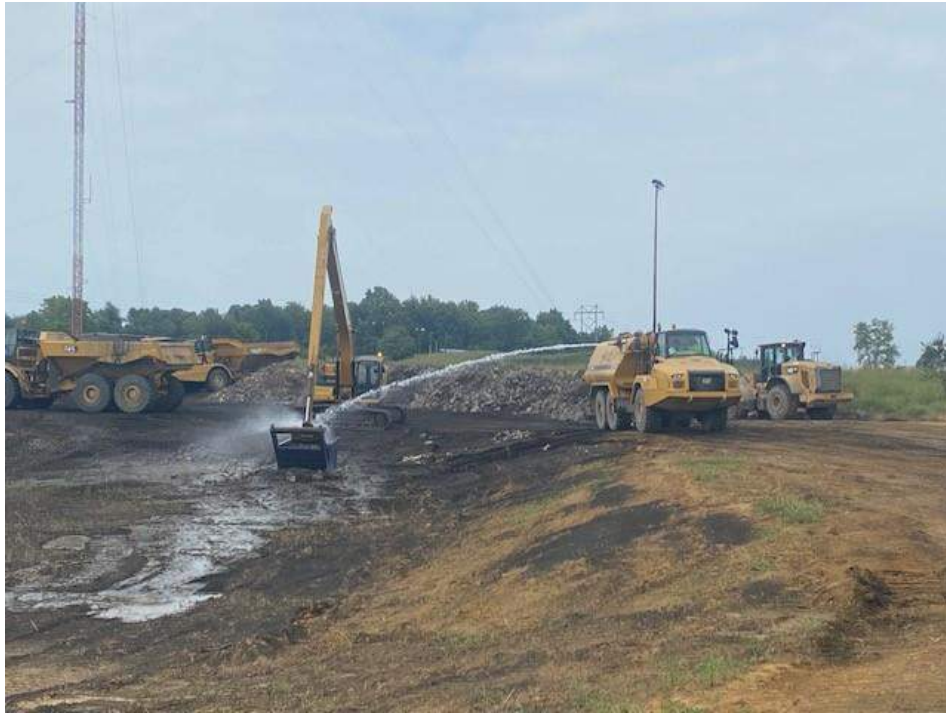
Photograph 3. Decontaminating and stockpiling riprap for reuse.
