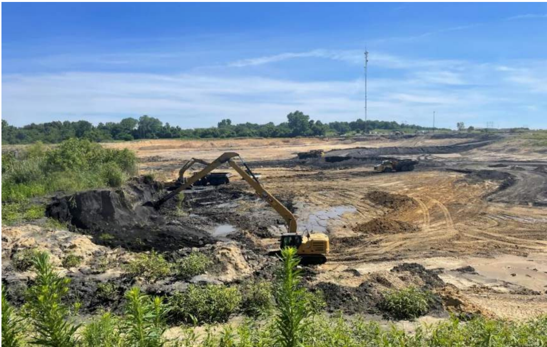
Photograph 36. Excavating ash prior to loading into haul trucks for transportation to landfill.
