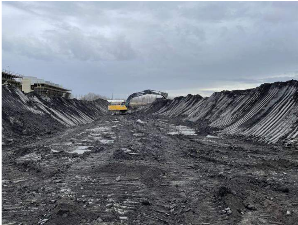
Photograph 13. Continued ash excavation. (Photograph taken by Charah Solutions, LLC, December 2023)
