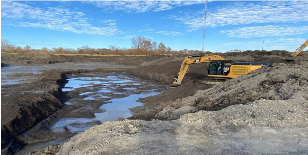
Photograph 9. Expansion of sump downstream of rim ditch. (Photograph taken by Charah Solutions, LLC, November 2023)
