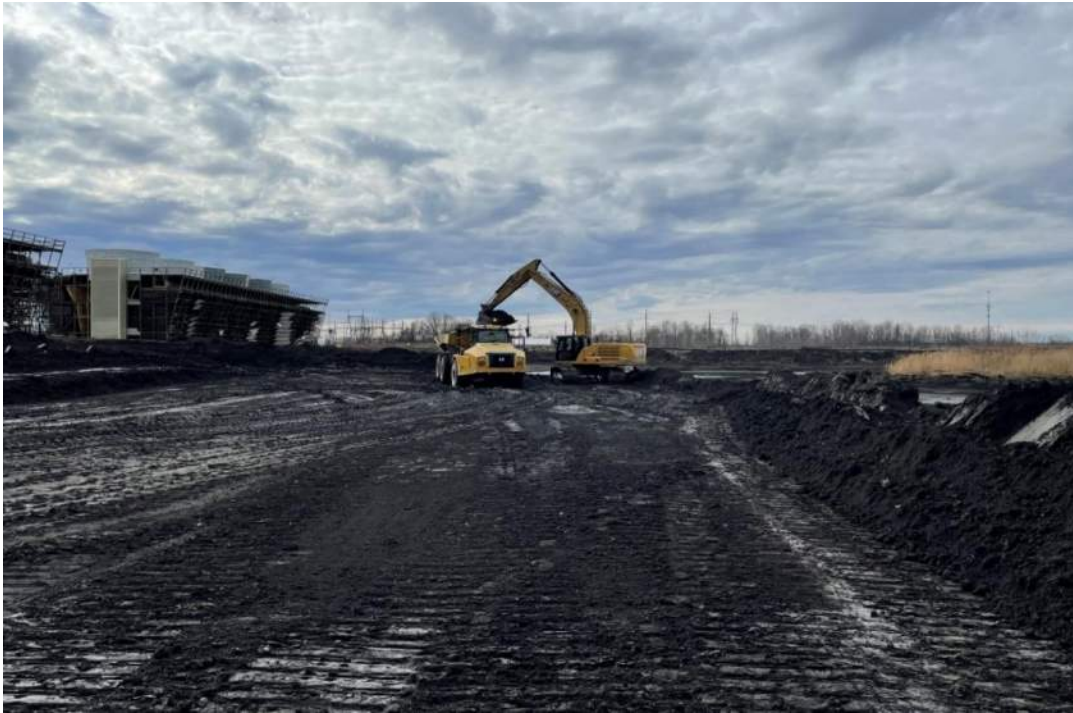
Photograph 15. Loading ash into haul truck for transportation to landfill.
