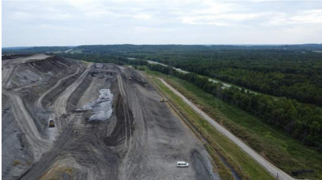
Photograph 40. Placing ash in Green Station CCR Landfill.
