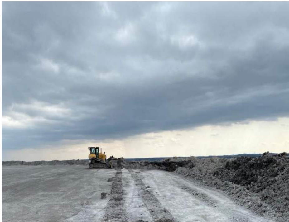
Photograph 22. Placing and grading ash in Green Station CCR Landfill. (Photograph taken by Charah Solutions, LLC, March 2024)
