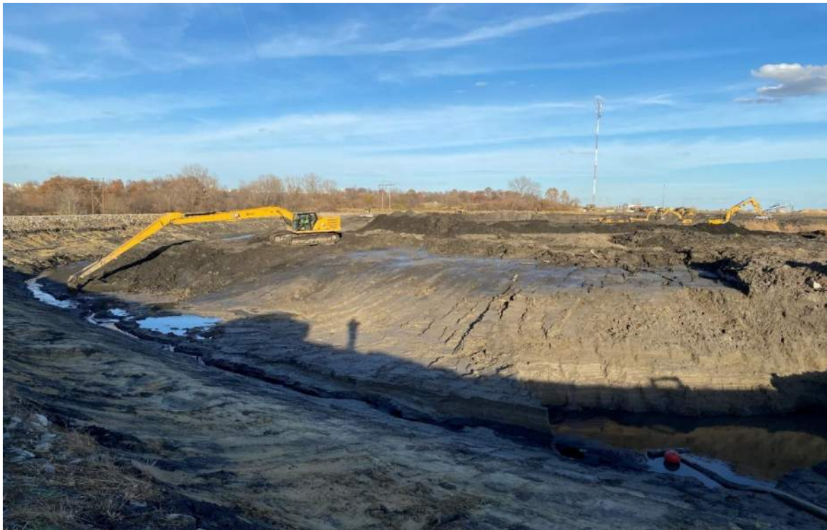
Photograph 11. Continued excavation of rim ditches to promote dewatering of impounded ash. (Photograph taken by Charah Solutions, LLC, November 2023)
