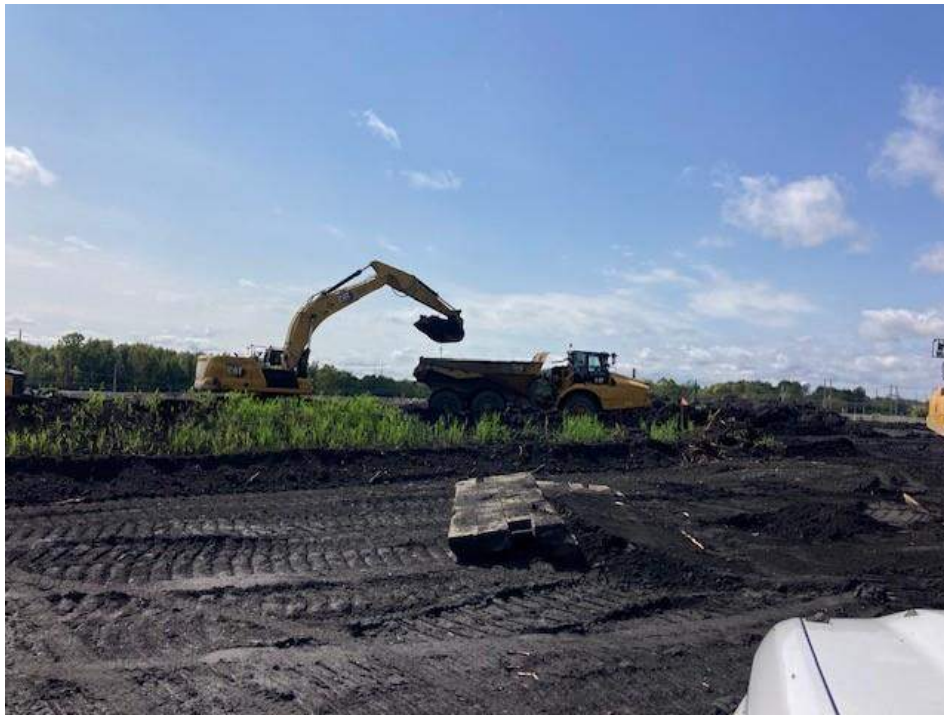
Photograph 5. Loading ash into haul truck for transportation to landfill.
