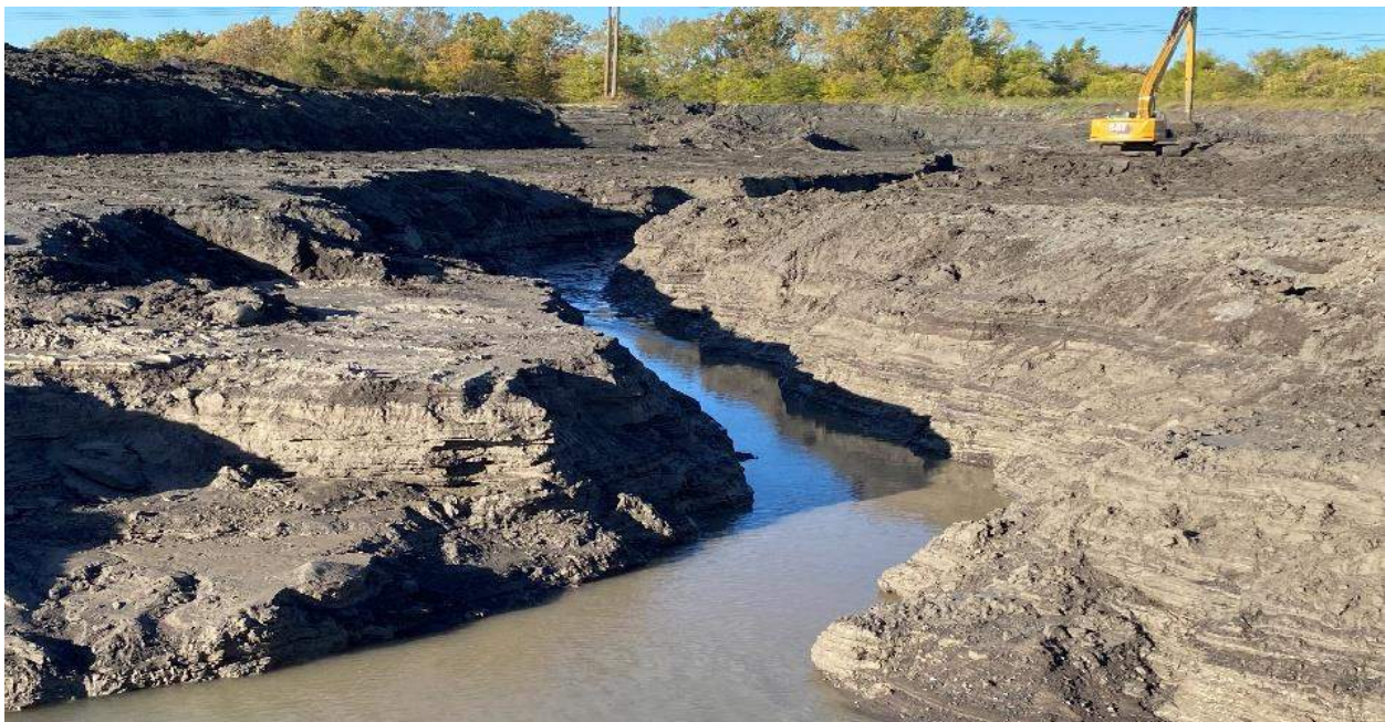
Photograph 6. Rim ditch to sump upstream of bulk dewatering system.
