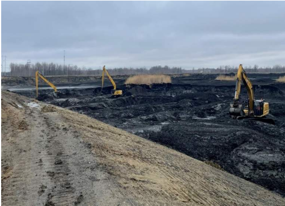
Photograph 21. Working ash within decant area / sump to promote dewatering. (Photograph taken by Charah Solutions, LLC, March 2024)
