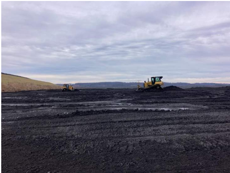
Photograph 16. Grading ash placed in Green Station CCR Landfill.
