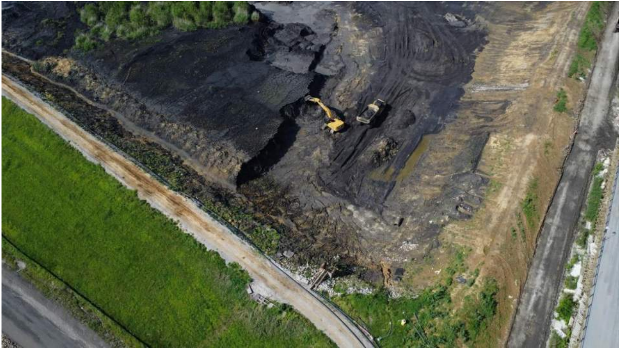
Photograph 27. Loading ash into haul truck for transportation to landfill.
