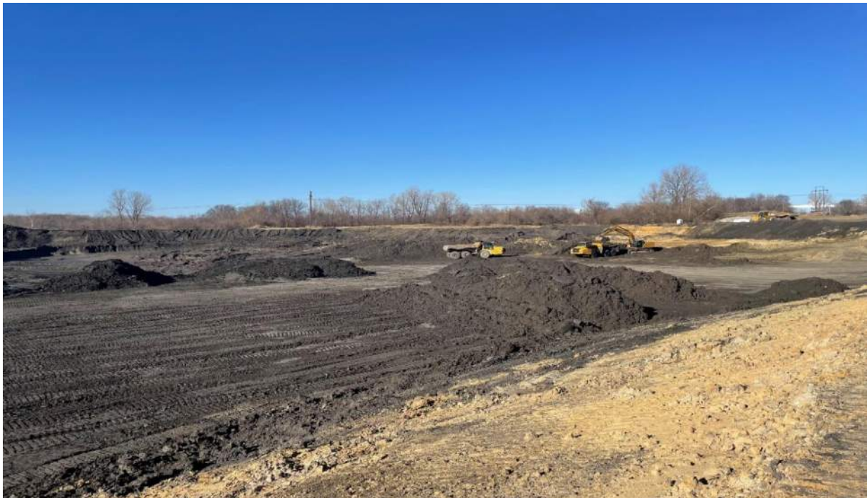
Photograph 20. Loading ash from decant area into haul truck for transportation to landfill.
