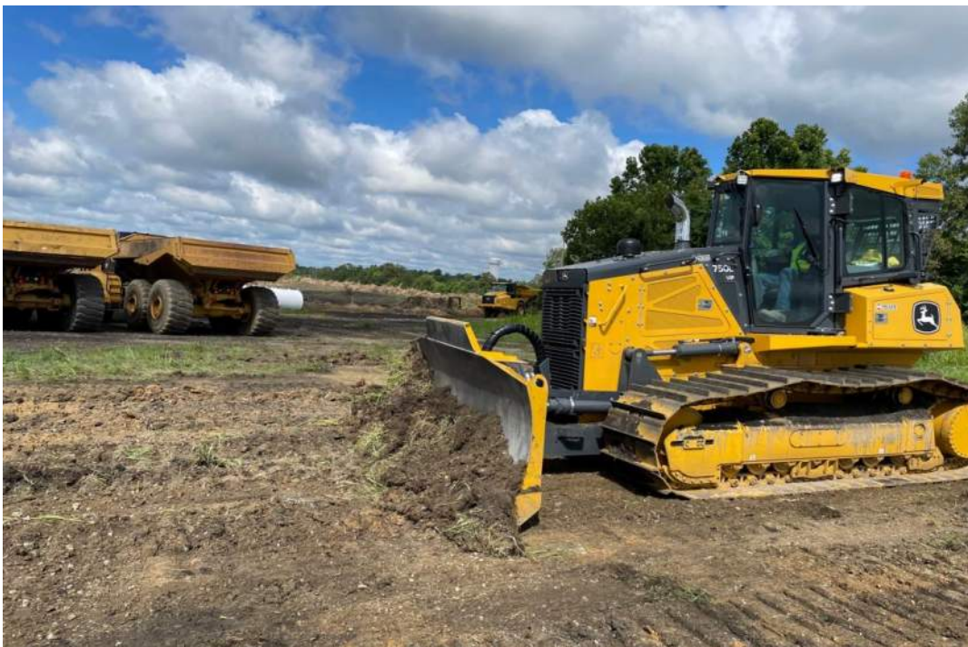
Photograph 2. Stripping vegetation and topsoil from impoundment area.
