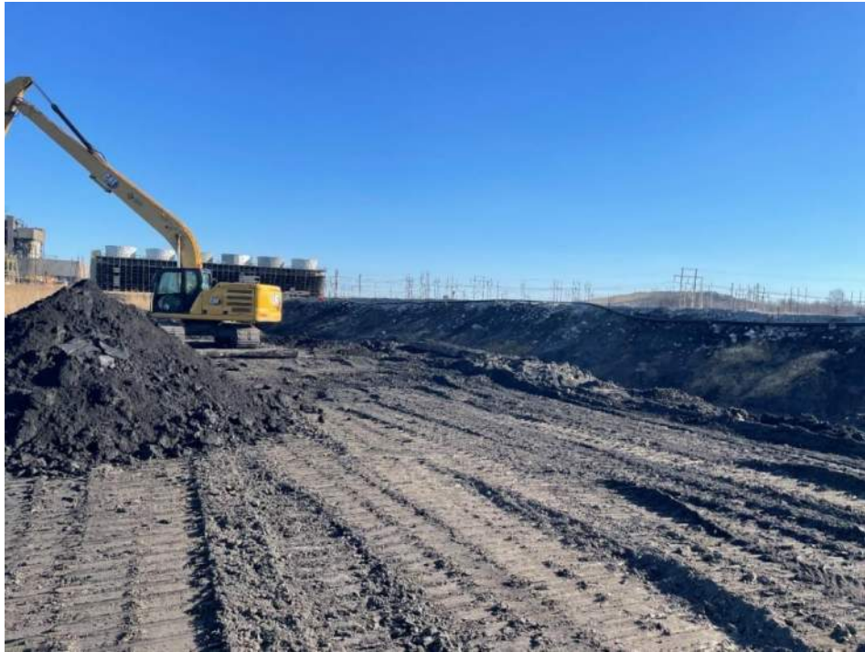
Photograph 19. Working ash within decant area / sump to promote dewatering.
