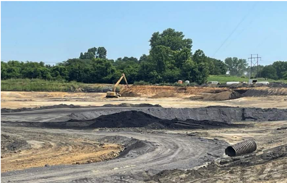
Photograph 33. Removing ash from impoundment berms. (Photograph taken by Charah Solutions, LLC, June 2024)
