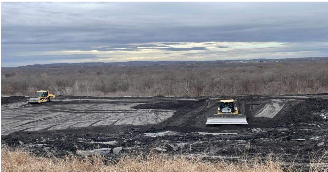
Photograph 12. Placement and compaction of ash in Green Station CCR Landfill. (Photograph taken by Charah Solutions, LLC, December 2023)
