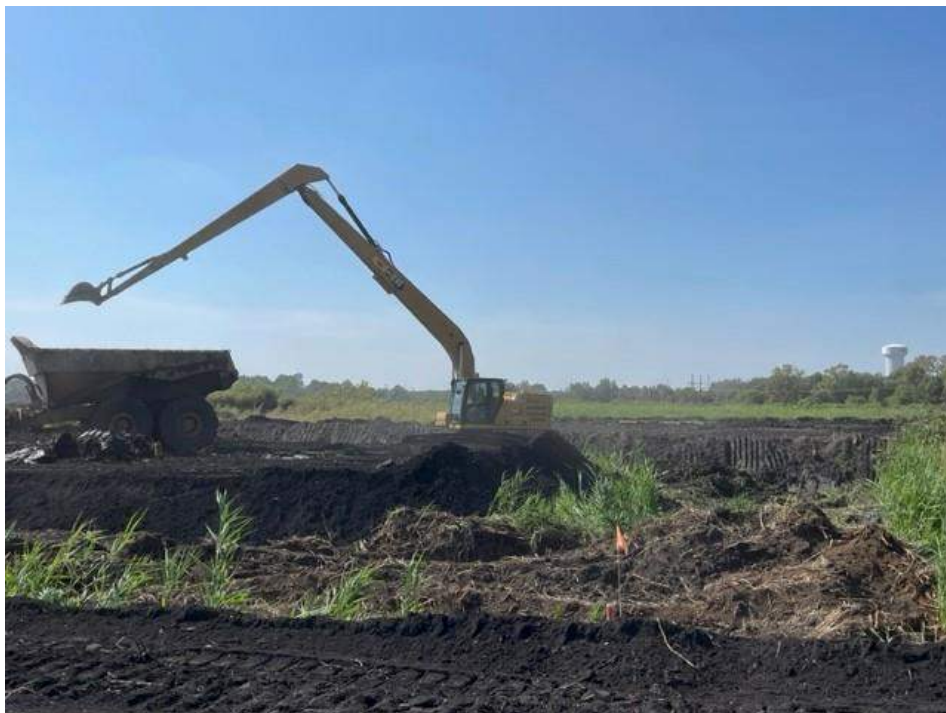
Photograph 4. Excavating rim ditches to promote dewatering of impounded ash.
