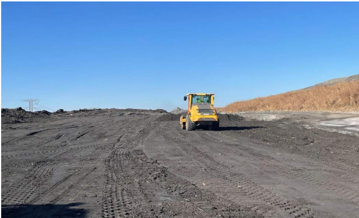
Photograph 10. Placement of ash in Green Station CCR Landfill. (Photograph taken by Charah Solutions, LLC, November 2023)
