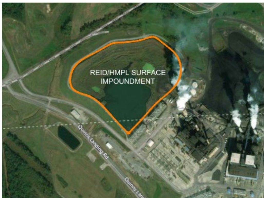
Figure 1: Big Rivers Reid/HMPL CCR Surface Impoundment Overview
