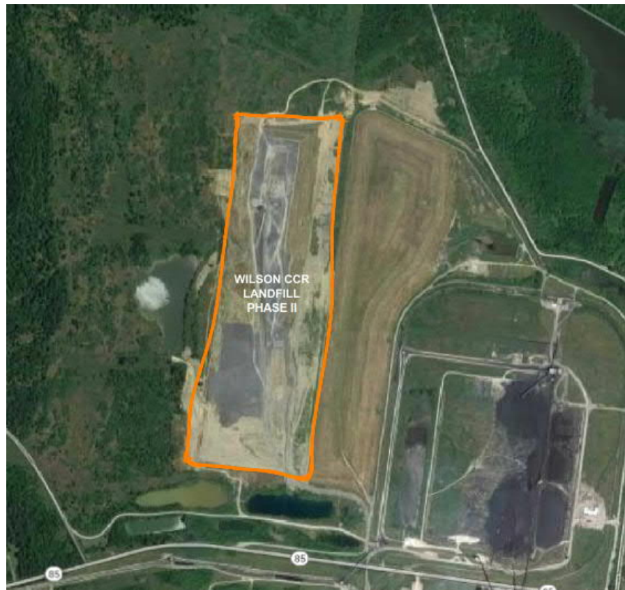
Figure 1: D.B. Wilson Phase II CCR Landfill Aerial Photograph
