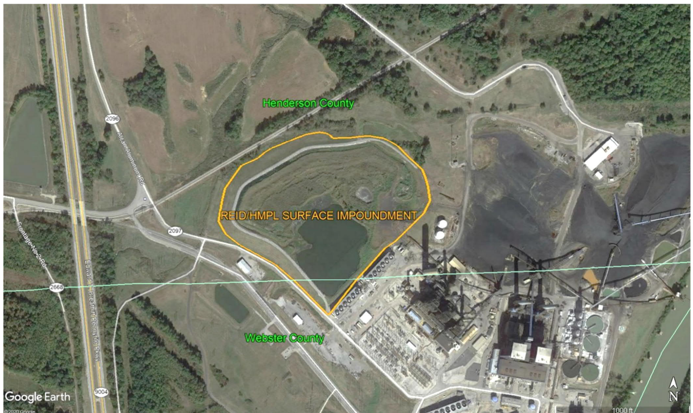
Figure 1: Big Rivers Reid/HMP&L CCR Surface Impoundment Overview (Google Earth, 2020)
