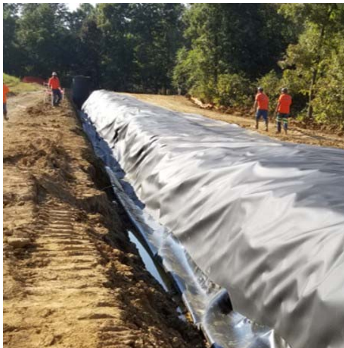
Photo 3: Installation of the Northwest Seep Collection Trench in September 2019.
