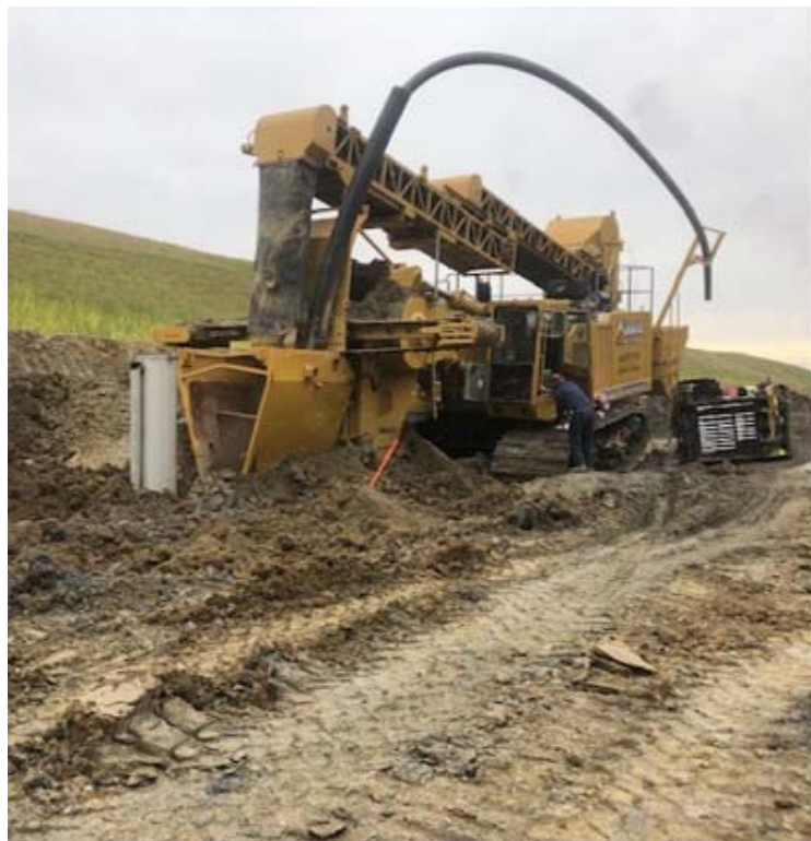
Photo 2: Installation of the Deep Seep Collection Trench in October 2019.
