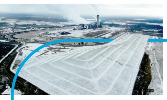
Big Rivers successfully closed the first phase of the Wilson Station Landfill using a groundbreaking synthetic liner and artificial turf system that prevents groundwater penetration and reduces annual maintenance costs.
